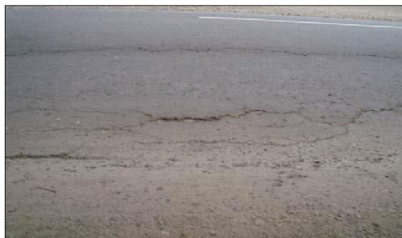
Gambar 2.4 Cekungan ( Bumb and Sags )
