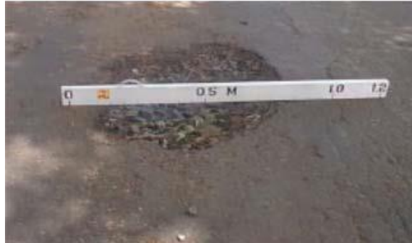
Gambar 2.13 Lubang (Pothole)
