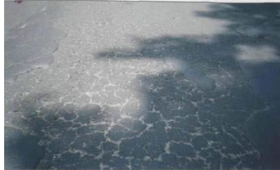
Gambar 2.19 Pelepasan Butir ( Weathering/Raveling )
