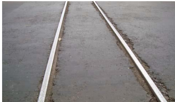
Gambar 2.14 Rusak Perpotongan Rel ( Railroad Crossing )
