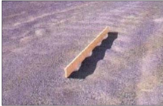
Gambar 2.5 Keriting (Corrugation) Sumber : Bina marga no.03/MN/B/1983
