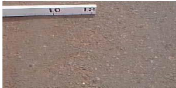
Gambar 2.12 Pengausan Agregat (Polished Agregat) Sumber : Bina marga no.03/MN/B/1983
